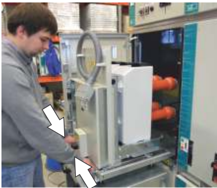
Slide 2 handles simultaneously to the middle
