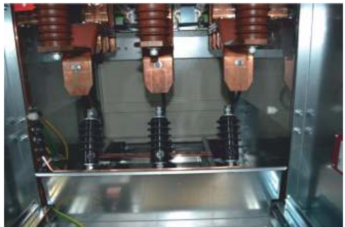
Fig.4.5. Auxiliary contacts of the earthing switch
