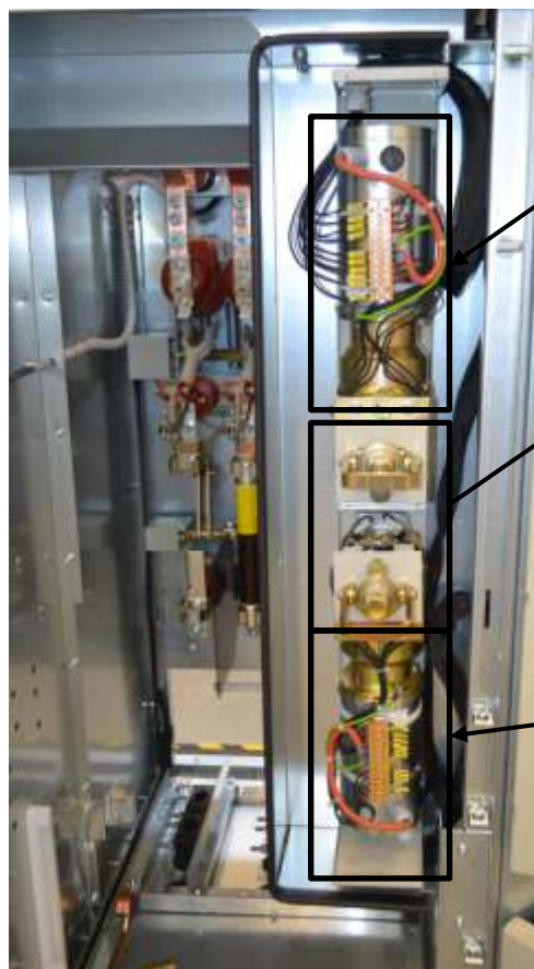
LBSF panel with motor operating devices inside
