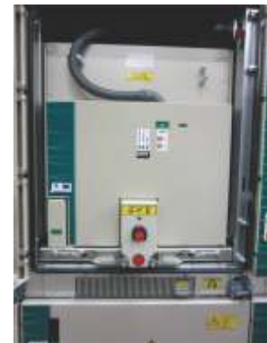
DOU is in the test position
