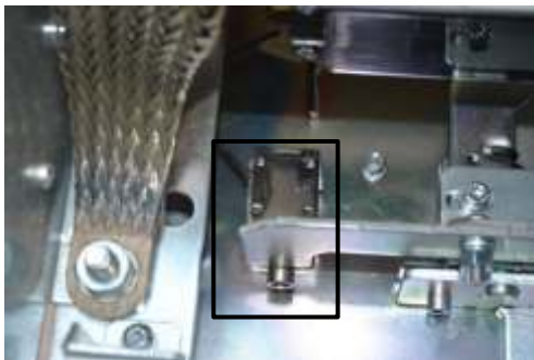
Position of activated interlock inside DOU (no voltage applied)
