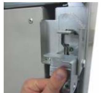
Socket for operation with earthing switch
