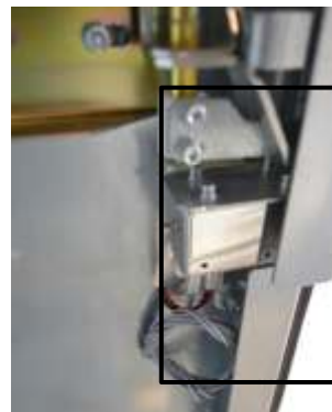
Earthing switch electromagnetic interlock
