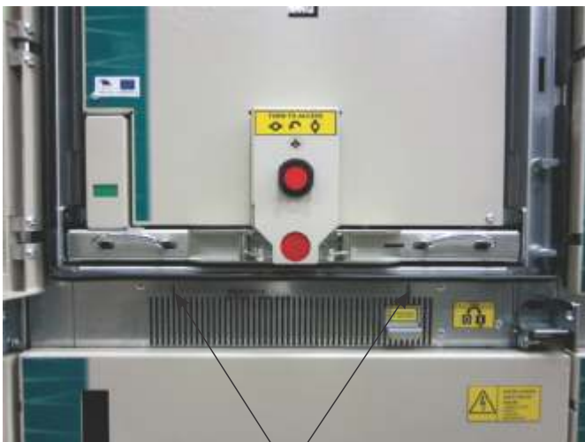
Openings for trolley guides
